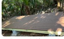
pads. It has been going well. I've worked for more than a month, and I, along with a couple of others working with me, have completed 8 so far. We start by leveling the ground, building the frame, then screwing in the decking boards. This project was put on pause due to the Mud Run, as I was helping build the obstacles. I still have 4 left to build which I'm hoping to finish before the summer Boot Camp program starts in mid-June.
